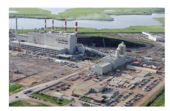
The BD3 CCS Facility began operation in 2014, a retrofit that extended the life of the Boundary Dam Power Station's oldest 150-megawatt turbine with a CCS retrofit designed to capture **90%** of the unit's CO<sub>2</sub> emissions.
