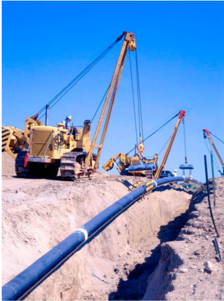
Figure 29. The CO 2 pipeline from Beulah, North Dakota, to southern Saskatchewan is buried more than six feet deep to minimise the potential for ruptures. (Photograph courtesy of Dakota Gasification Company)
