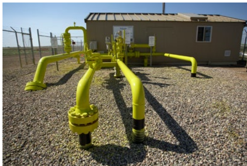
Figure 6. Here, the CO 2 at the Weyburn oilfield is pumped to various locations in the field for injection underground. The yellow indicates the pipelines are transporting CO 2 . (Photograph courtesy of Cenovus Energy)
