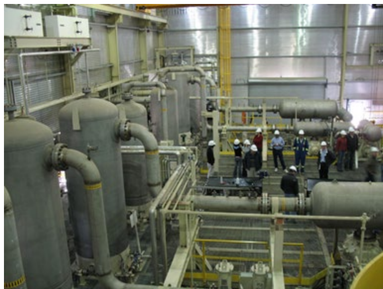
Figure 4. These compressors, at the Dakota Gasification Facility in North Dakota, condense the \text{CO}_2 into a “dense phase” so that it will flow like a liquid in the pipeline to Canada. (Photograph courtesy of Dakota Gasification Company)
