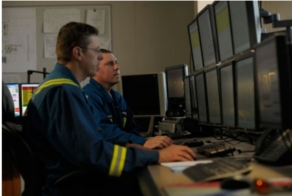
Figure 28. Staff at Cenovus's Weyburn oilfield monitor CO 2 pipelines using computers with advanced pressure and temperature technologies. (Photograph courtesy of Cenovus Energy)
