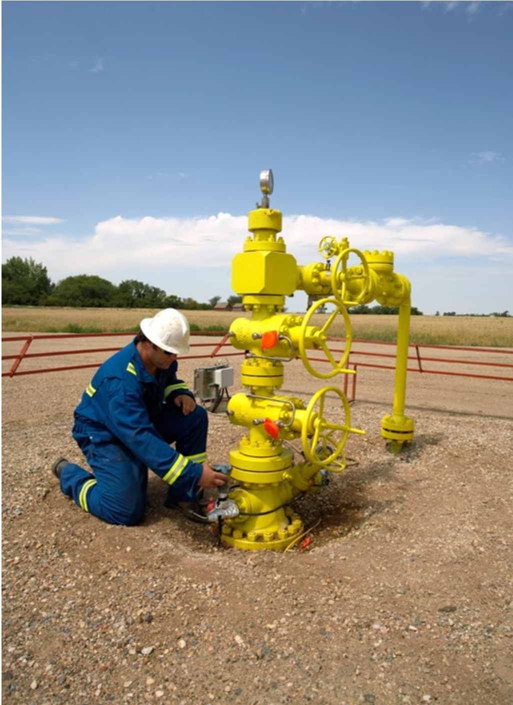
Figure 21. This CO 2 injection well has a wellhead that can be turned off, stopping injection. Wellbores that are not currently producing oil or being used for injection will have a wellhead such as this on the surface. Wells that are no longer in use will have their wellhead removed and will be cemented down the full length of the wellbore to ensure they do not allow for the upward movement of liquids and gases. All surface lines and equipment will be removed and the well will be permanently capped. (Photograph courtesy of Cenovus Energy)
