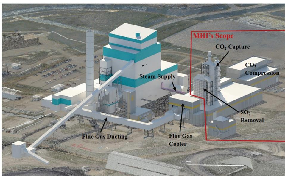
Figure 1. 3D model of the proposed CO<sub>2</sub> capture facility for the Shand power station.**Table 3. Shand's current operating performance.**
