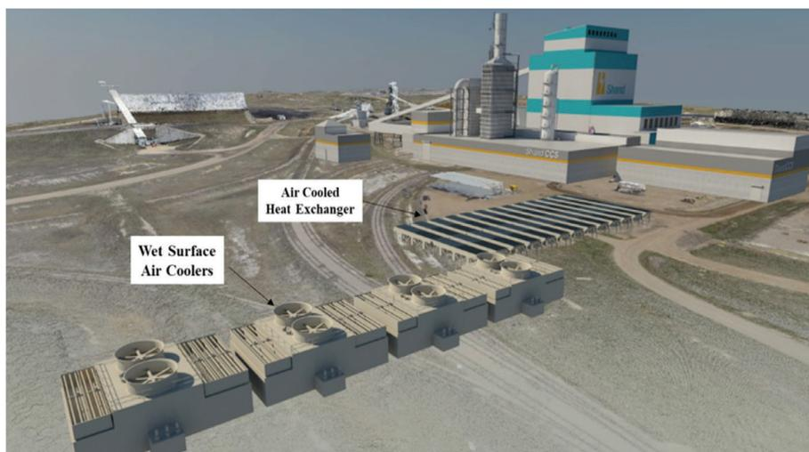
Figure 6. Proposed Shand hybrid cooling system.
