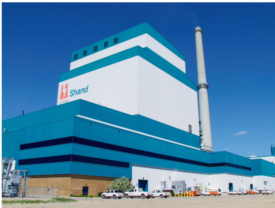
A feasibility study is being conducted on retrofitting SaskPower’s Shand Power Station for post combustion carbon capture
