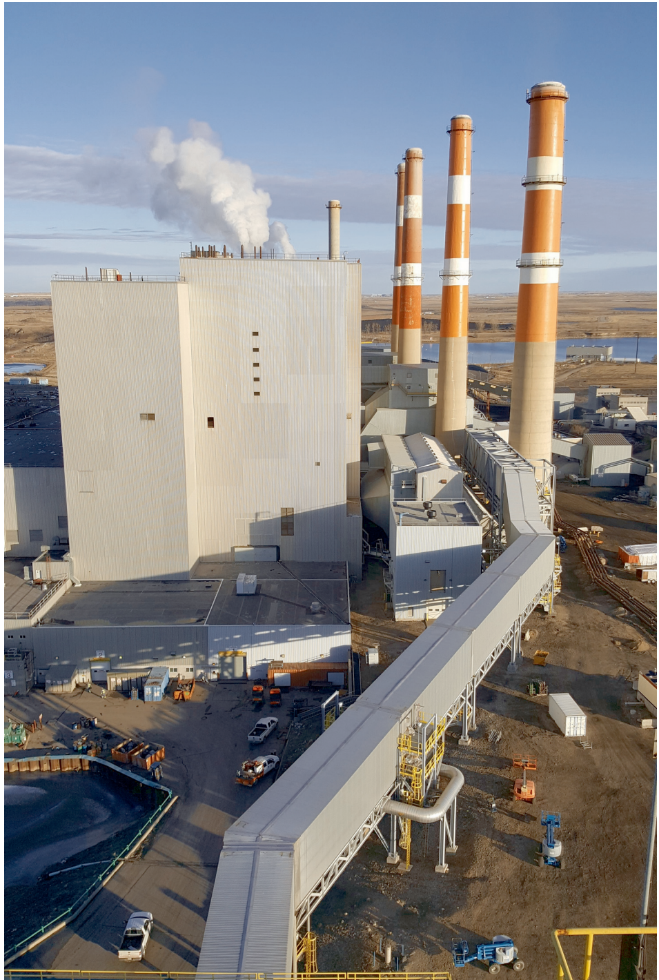
Work on SaskPower's Boundary Dam 3 CCS Facility (BD3) is now focussed on optimising the facility and knowledge gained will be used to inform the Shand feasibility study
