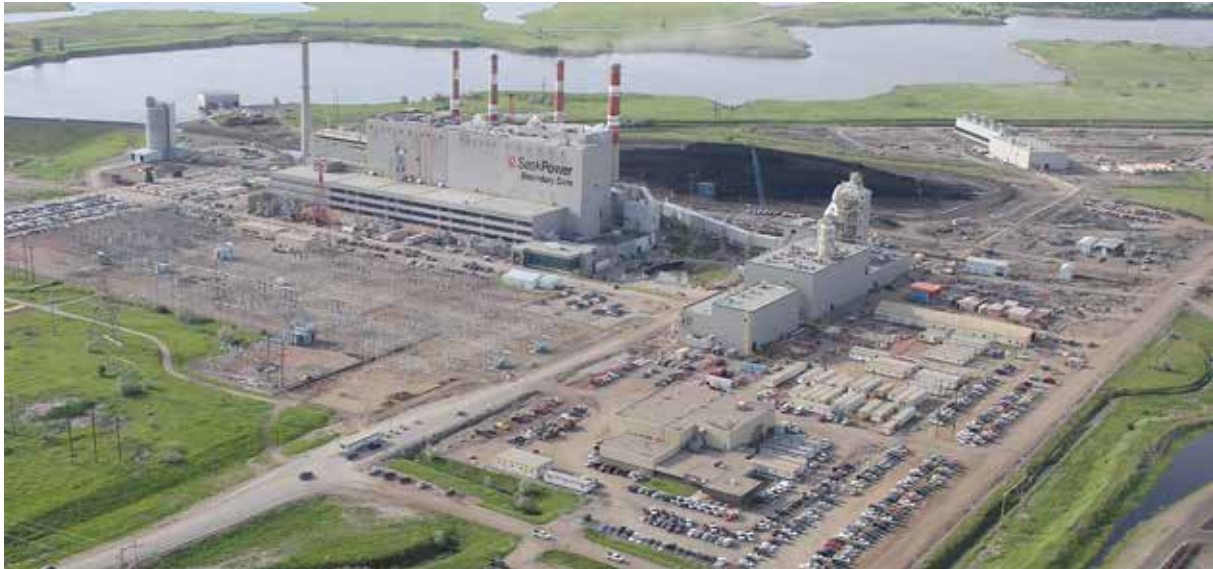
Aerial View of the BD3 Capture Facility at the SaskPower Boundary Dam Power Station located near Estevan Saskatchewan (Courtesy: International CCS Knowledge Centre).
