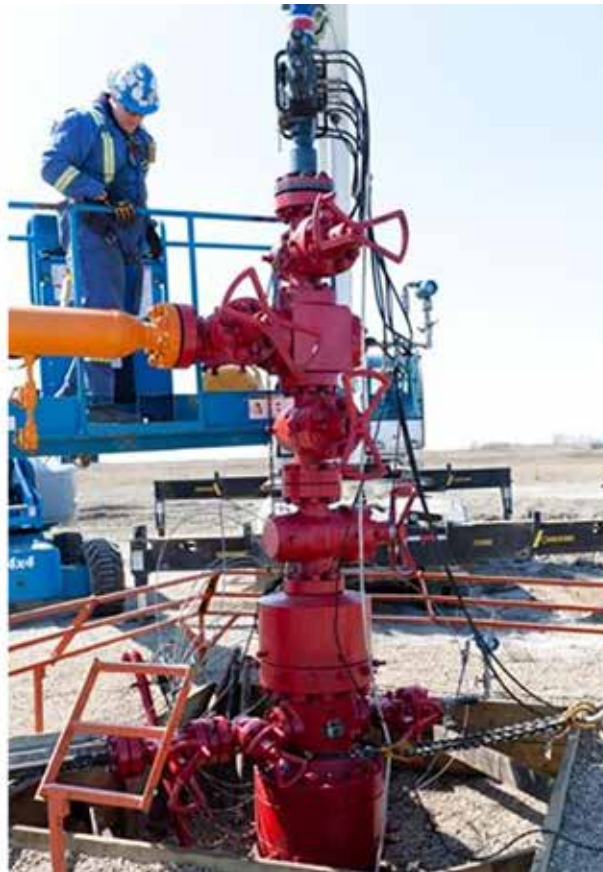
The Aquistore injection well during its installation (Courtesy: Petroleum Technology Research Centre)
