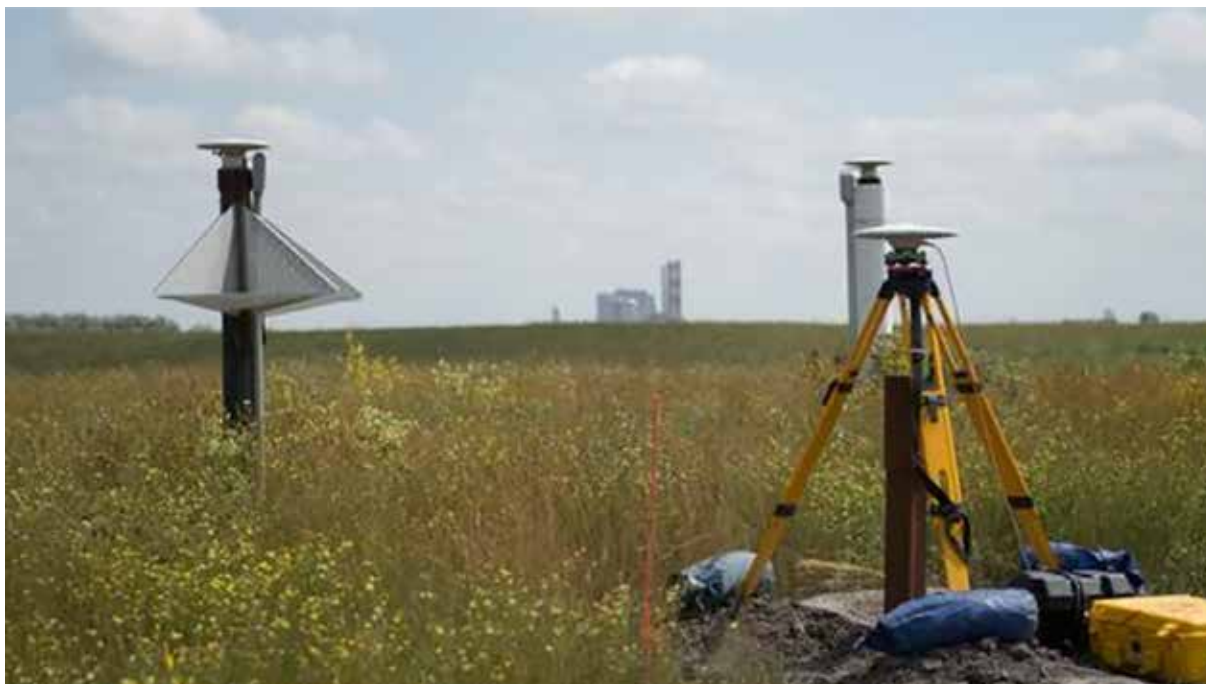
Surface monitoring equipment at the Aquistore CO 2 storage site. The BD3 Carbon Capture Facility (in background) sends CO 2 by pipeline for injection deep underground (3.4 km) and permanent storage (Courtesy: Petroleum Technology Research Centre).
