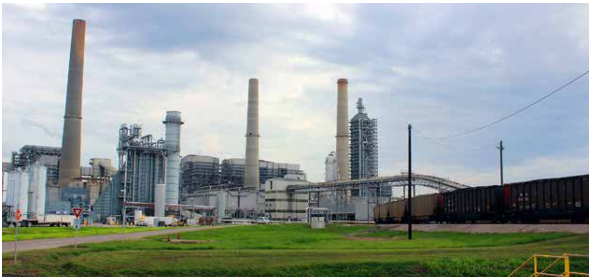
Carbon Capture Facility at Petra Nova WAParish Station, (Courtesy: NRG Energy).
