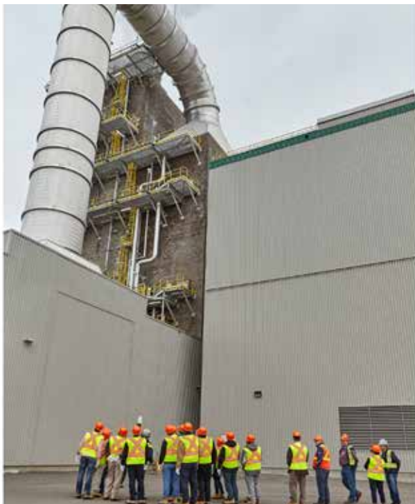
A tour group at the BD3 Carbon Capture Facility (Courtesy: International CCS Knowledge Centre).
