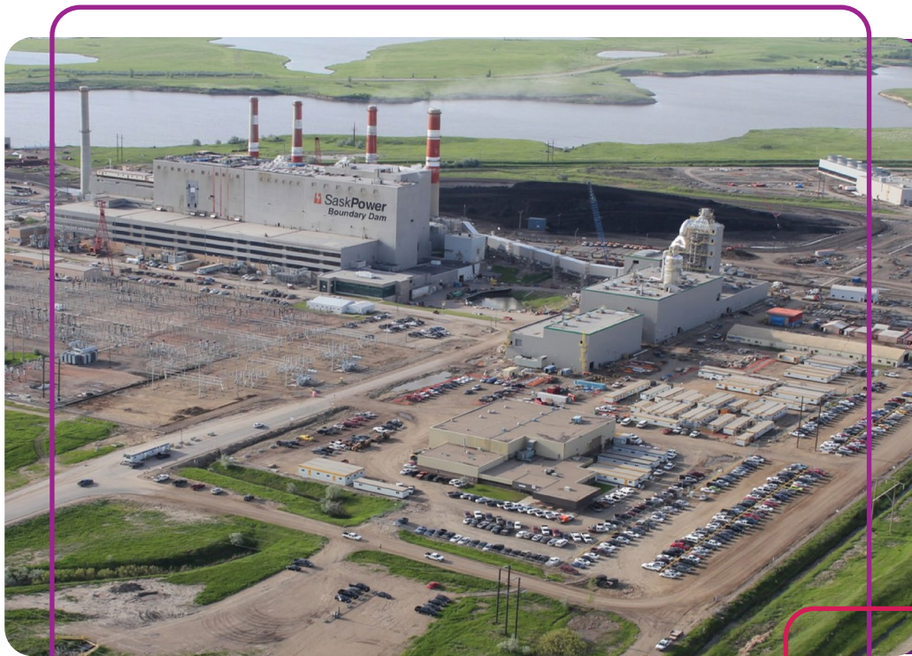
Aerial view of the BD3 Capture Facility at the SaskPower's Boundary Dam Power Station located near Estevan, Saskatchewan
